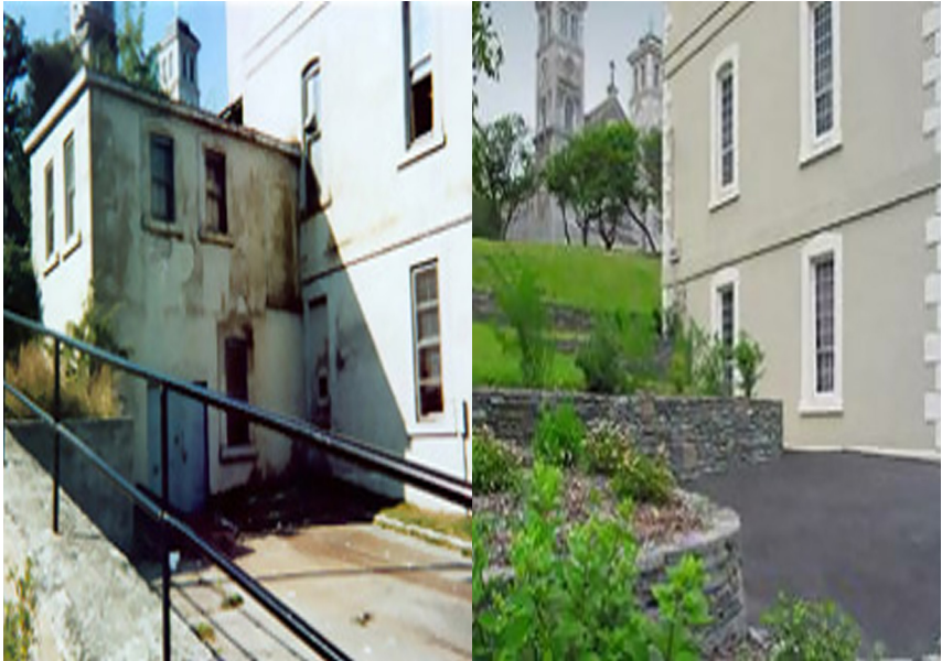
Above: Before and after photos of St. Patrick's Hall (1877) fully restored by Kevin Nolan and Robert Hall (2002)
